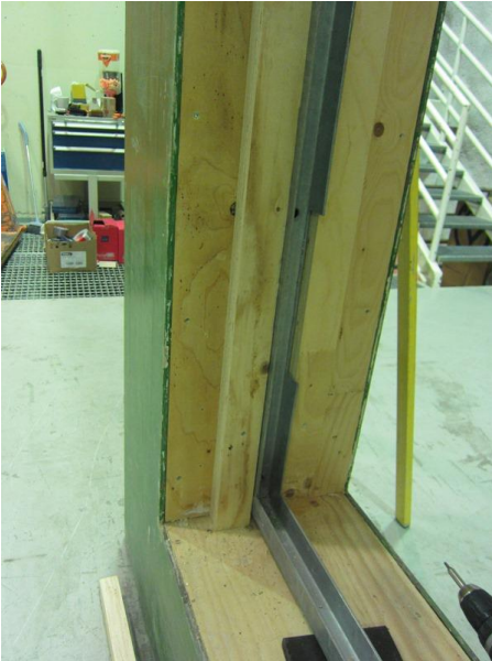
Photo 1. Steel frame for installation of planks to test opening
