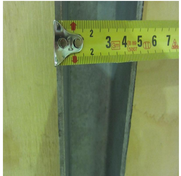
Photo 2. Steel frame thickness
